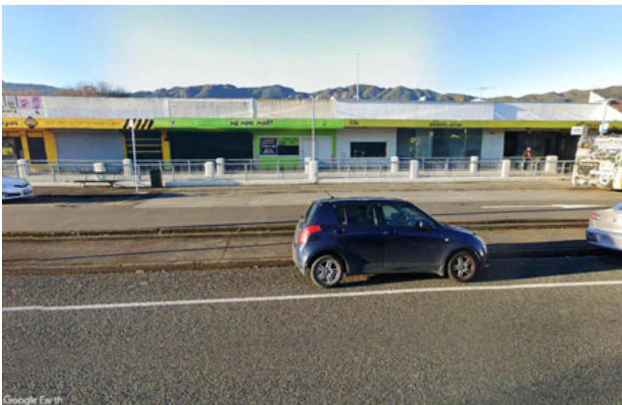
Figure 8 . Buildings with “fronts” facing Cambridge Terrace.
