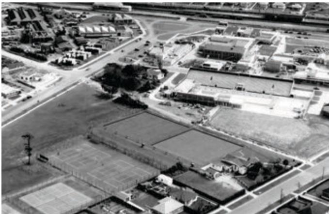
Figure 17. Aerial photograph from 1958 showing the Naenae swimming pool under construction.
