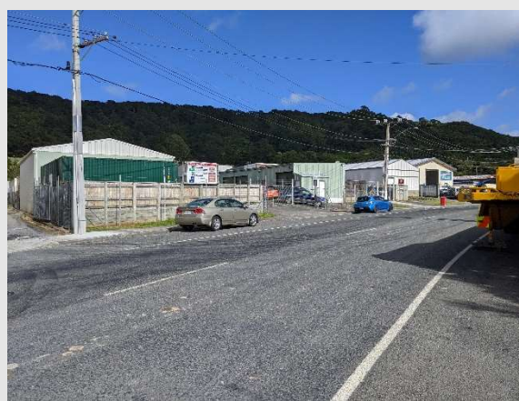
Photo 10: Buildings east of Waiu Street. Two companies, Wainui Self Storage and Auto Maintenance and Marine, are visible.
