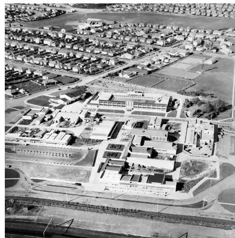
Figure 5 - Naenae town centre under construction. 1958.
