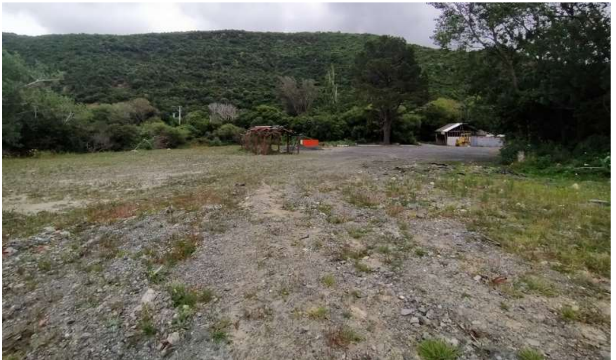
Figure 11 South end of development area- showing heavy machinery disturbance (25 th January 2022).
